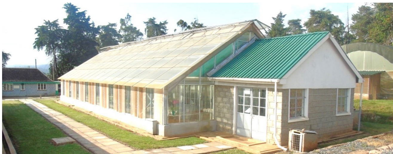
Plant Quarantine & Biosecurity station has quarantine greenhouse and screen house facilities for carrying out biological assays, grow out tests as well as for maintenance of reference material e.g. viruses on live plants
